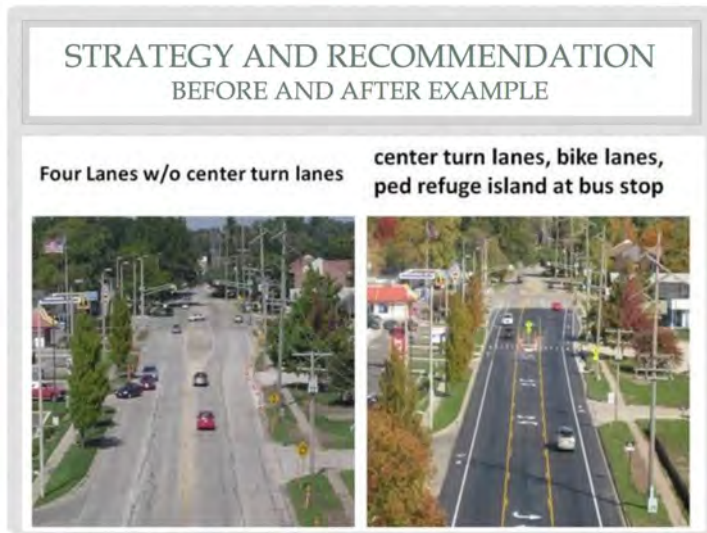
Page from the BCA Arterial Roads Sidewalks and Pedestrian Safety Task Force presentation showing example configuration option for Wilson Blvd.
